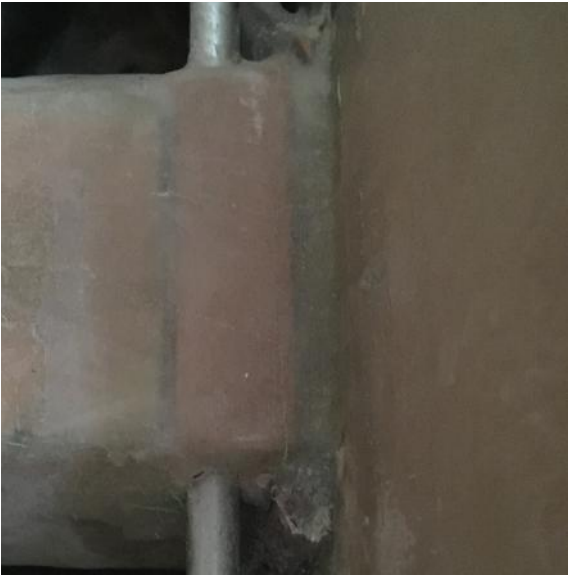
Figure 11 Completed central tunnel slot closure
