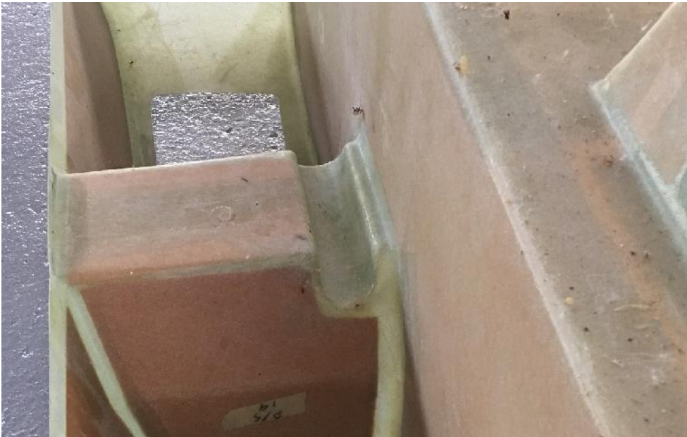
Figure 6 Photo of the preformed slot
