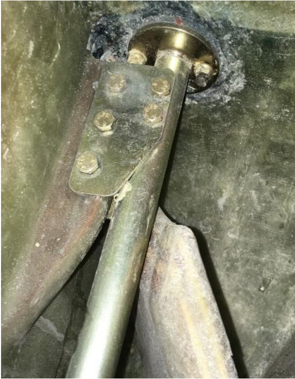
Figure 8 Final installation of gusset plates
